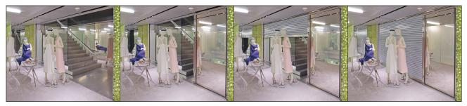
T2000 Series fire door assemblies incorporate either one or two deployable egress doors which are flush mounted in an adjacent wall. Upon activation by a building alarm or in an emergency condition, these complying egress doors swing into position. The doors then serve as side guides for the vertical coiling door assembly as it descends to provide complete protection from fire and smoke, and provide conventional egress as required.
