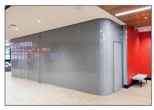
This bi-parting \$7902 with two integral swing doors negotiates two 18" radius curves to create a complying interior exit stairway shaft enclosure.
