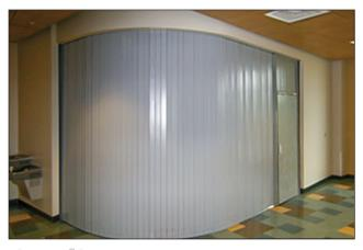
Incorporating conventional egress swing doors with fire exit hardware, the Safescape® \$9000 fire door can easily negotiate a 3' radius curve.
